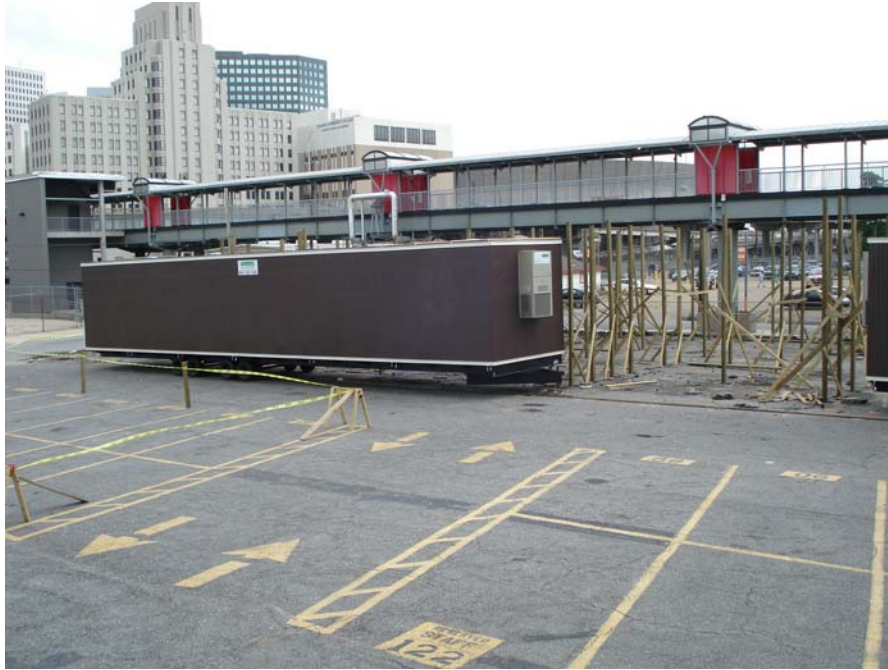
Trailers have arrived and the construction of the center is underway
